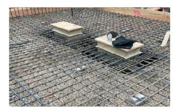
Floor rebar being installed around pool drains in deep section
